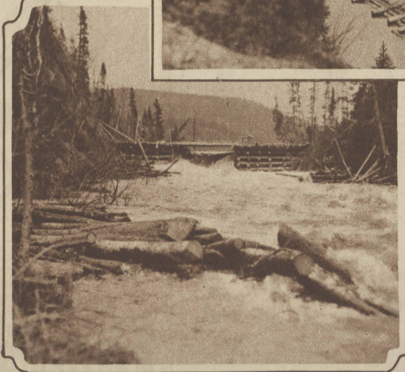
DAMS CONSERVE WATER NEEDED FOR "DRIVE" —After the spring floods many rivers, if left to themselves, would soon become shallow rivulets. To prevent this The Tribune builds dams behind which the needed water is conserved. They are opened only to permit the passage of logs.
