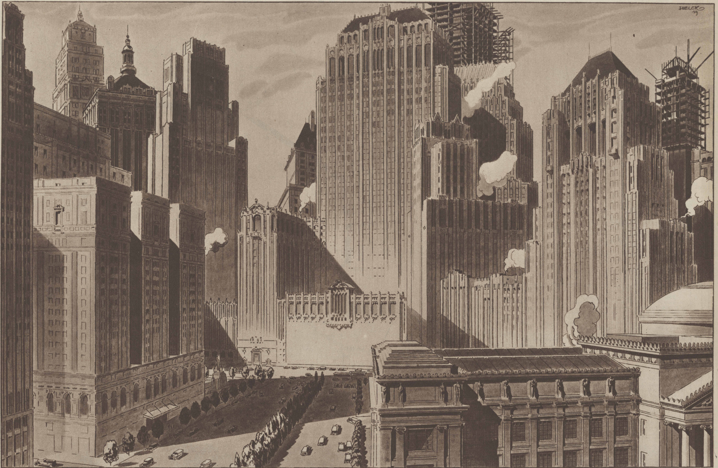
These buildings are electrically equipped entirely or in part by Westinghouse. From left to right: Eaton Tower, Detroit; Ritz Tower, New York; New York Central Building, New York; Greater Wm. Penn Hotel, Pittsburgh; Harriman Nat'l Bank, New York; Savoy Plaza Hotel, New York; Civic Opera House, Chicago; Sir Francis Drake Hotel, San Francisco; Koppers Building, Pittsburgh; Fisher Building, Detroit; Brooklyn Museum of Art, Brooklyn.
