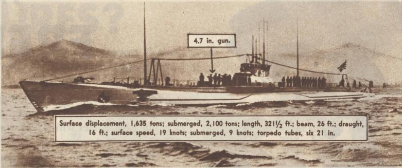
Associated Press photo CAPABLE OF A ROUND TRIP ACROSS THE PACIFIC without refueling are Japan's newer submarines. Some of the Japanese submersibles built since the 1-61 (pictured) carry two 4.7 inch guns; some mount eight torpedo tubes; and most of them are faster.
