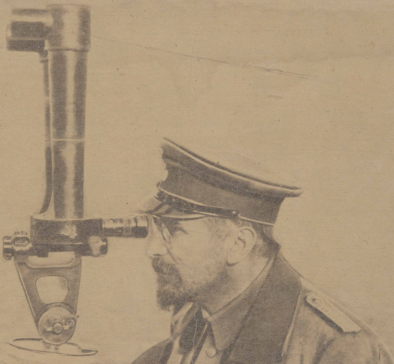
A German artillery officer directing the firing on Reims. His professional air well reflects the scientific business that war has become. The instrument is a combined binocular periscopic range finder. The wires of a field telephone appear overhead.
