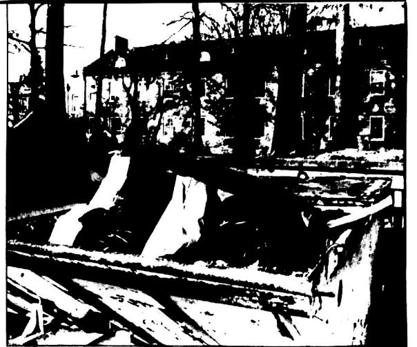
Garbage overflowing from receptacles behind Hillcrest Village Apartments is in violation of East Lansing housing code. Below, Ken Goodrich walks on a broken, chipped sidewalk, also a violation.
