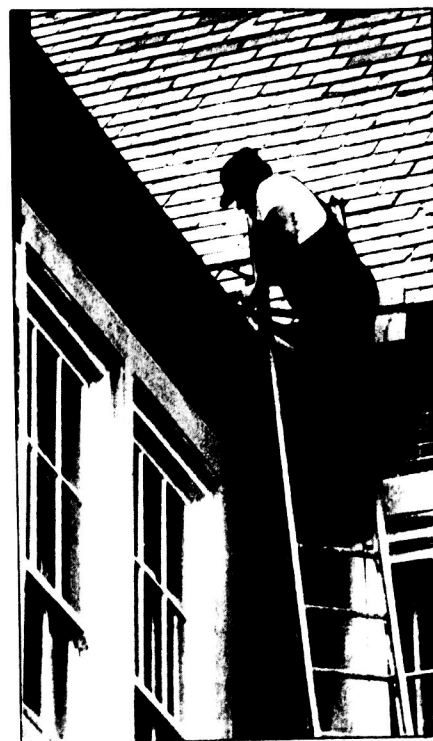
State News Deborah J. Borin There is no room for acrophobia in Dave Cook's business. Cook helped repair the loose slate shingles on the roof of the Natural Science Building.
