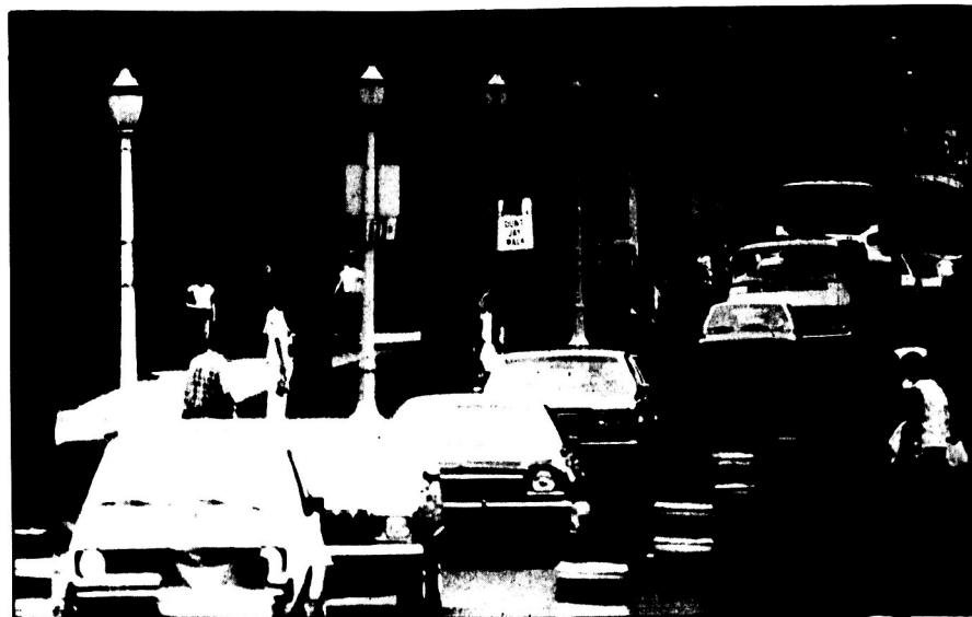
The Grand River Avenue congestion which began in July won't be getting less hectic, especially since the local population has doubled since the project began. Construction officials originally predicted that construction would be completed by the first MSU home football game this weekend.
