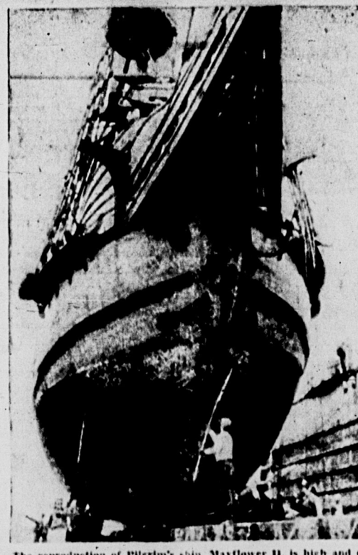
The reproduction of Pilgrim's ship, Mayflower II, is high and dry in Brooklyn drydock in New York with workers starting to scrape and paint its bottom. The vessel, which arrived in U.S. in June, has been on display in New York for the past four and one-half months. The 92-foot, 190-ton ship is being prepared for voyage to Plymouth, Mass., where it will be turned over to the Plymouth Foundation on Thanksgiving Day as a gift to America from the people of Great Britain.
