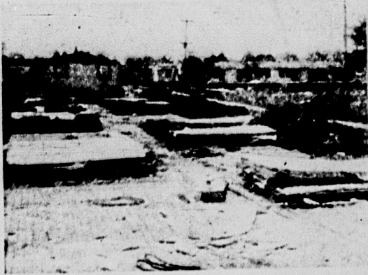
. . . the walls come tumbling down . . .
