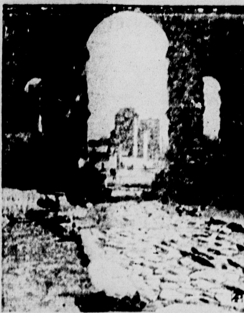
Street excavations for the enlargement of the Porta Maxima in Rome brought to light this stretch of an ancient road built in the reign of Marcus Aurelius.
