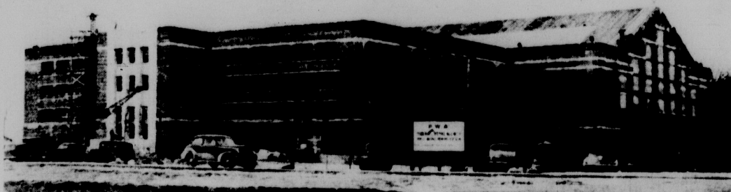
Although Jenison fieldhouse in general is far from completion the fieldhouse proper which occupies the western part of the building is far enough advanced to permit the playing of the State-Tennessee Basketball game there Saturday night.
