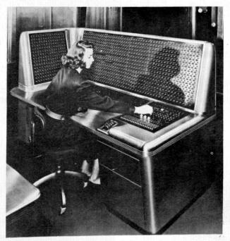
This machine is known as the console, or operation indicator and control desk for the IBM calculator.
