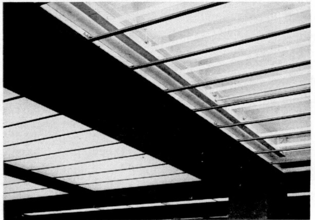
Shown here is a view of the ceiling in the assigned reading room of the new library. A portion can be seen where the plastic ceiling has been installed in contrast to that section that has been left bare. This is an illustration of one problem encountered by engineers working on the building.
