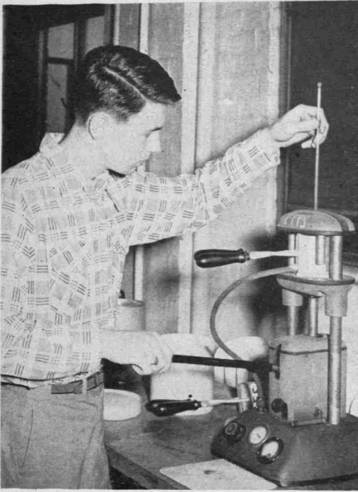
3. The two samples are mounted in clear bakelite.
