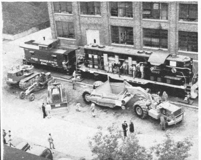
View in front of Shops building. Excavating equipment is in the foreground, while in the background is a Diesel switching engine and way car.
