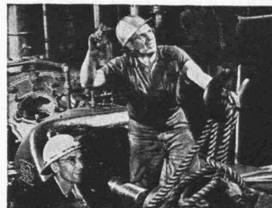
Keeping compressors in top running condition is a typical maintenance-group problem.
