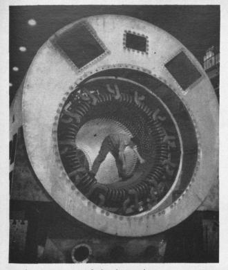
Inspecting one of the first turbine generators to be insulated with Thermalastic.
