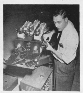
A view of the color camera showing the color separation setup. Each tube takes a one color image.
