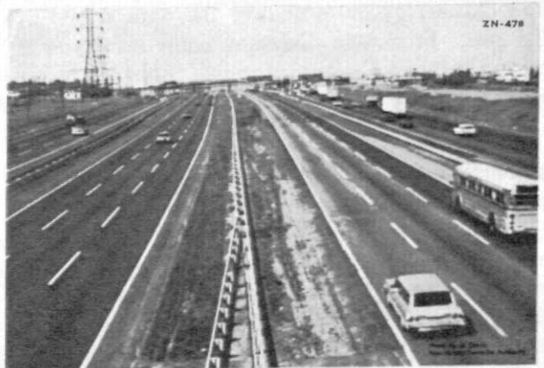
Galvanized steel guard rail on the New Jersey Turnpike has a record of no passenger vehicle breakthrough and no maintenance after ten years.
