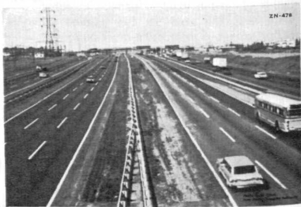
Galvanized steel guard rail on the New Jersey Turnpike has a record of no passenger vehicle breakthrough and no maintenance after ten years.
