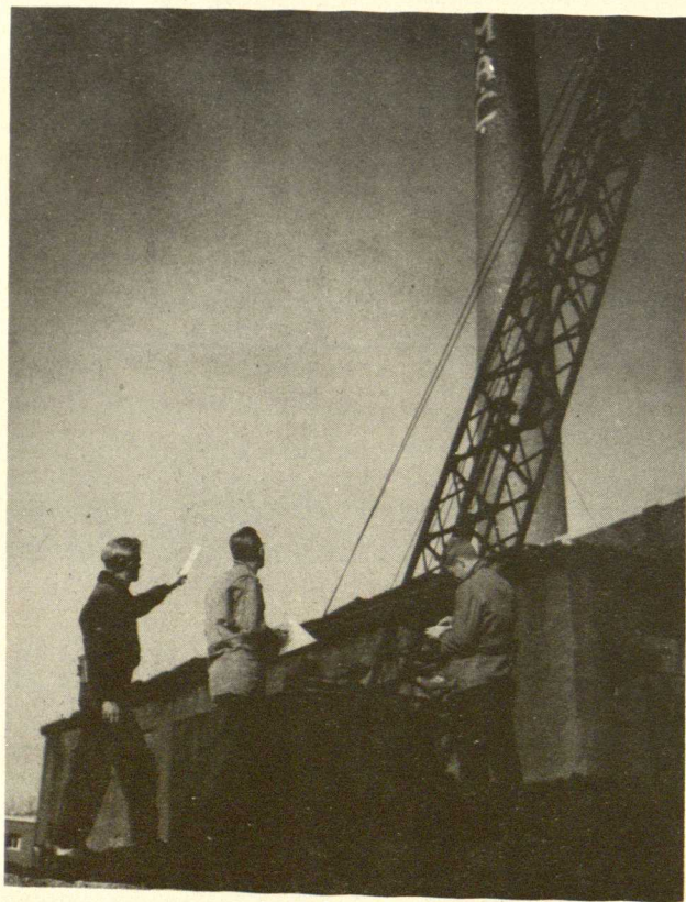
This view shows the many advantages of MSC's "huge" coal pile as a location for a Spectator Engineering Society meeting.
