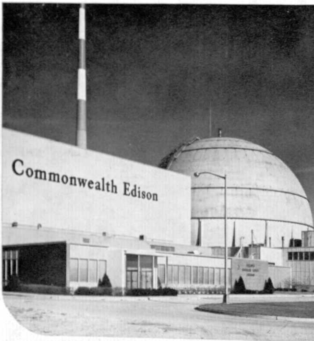
ELECTRIC UTILITY —Built by G.E., the Dresden Station produces commercial electric power from the atom.
