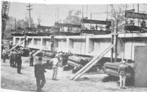
Pre-stressed Concrete Test Girder
