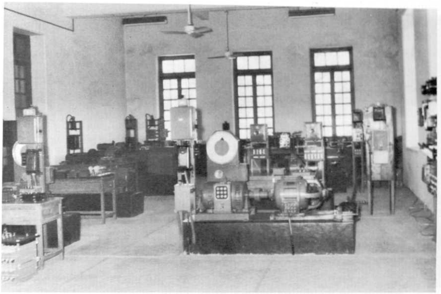
Motor-generator laboratory in Electrical Engineering Department, Engineering College, Poona.
