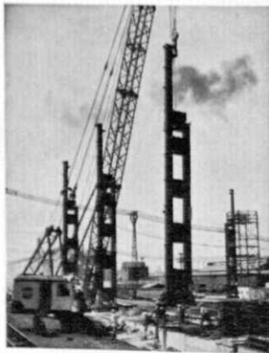
Installing new oxygen steelmaking furnaces at Lackawanna, N. Y.
