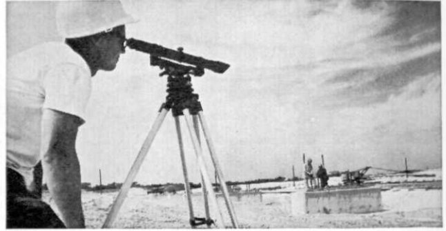
Building a $250-million steel plant at Burns Harbor, Ind.
