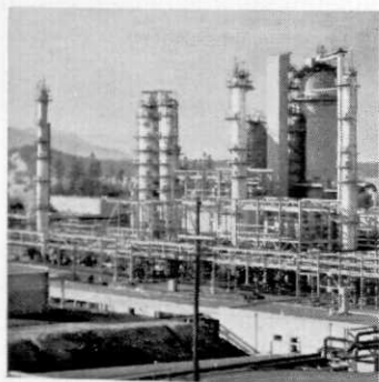
PROBLEM: Improve the reliability and precision of automatic controls and new materials and equipment demanded by new oil and chemical processes.
