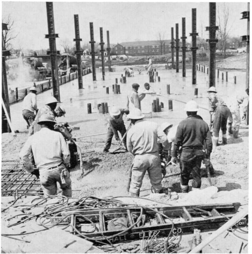
Workers smooth surface of ground floor.
