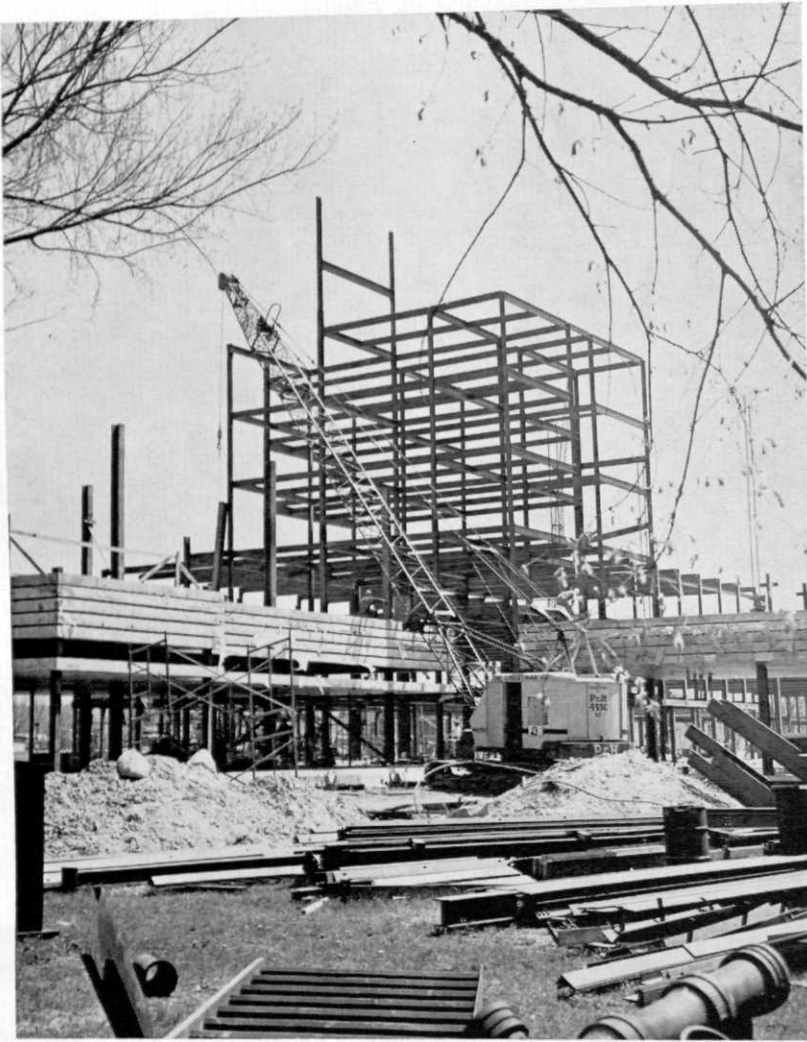
Case floors are poured and ready for lifting.
