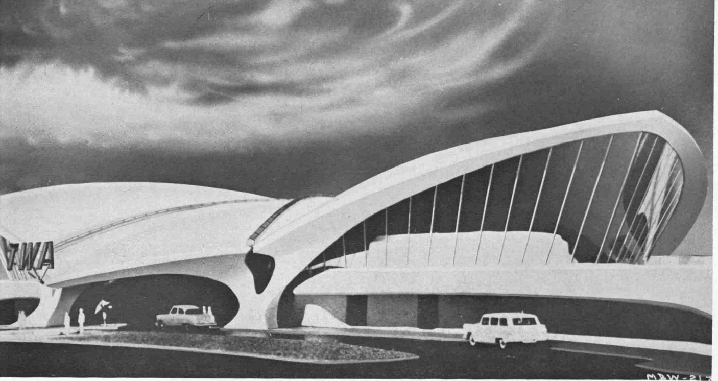
Model of the new terminal at Idlewild Airport to be completed in late 1961.
