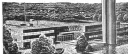
East Coast Laboratory and Microwave Tower
