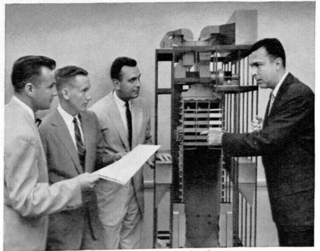
B&W engineers discuss developments in the Universal Pressure Boiler.
