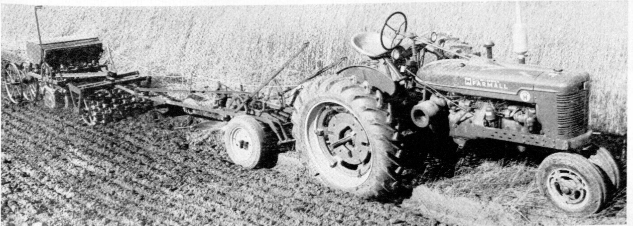
Illustrated is a true once-over tillage operation. The press-wheel drill is attached to the plow-packer, which is in turn attached to the plow.
