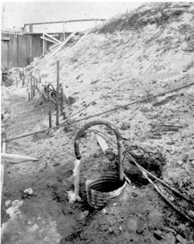
WELLPOINTS serve as cathodes, through which water escapes from the fine-grain silt, pushed out by electric potential. Header system has been removed, and water dribbles out of open-top wellpoint, freezing into an icicle.
