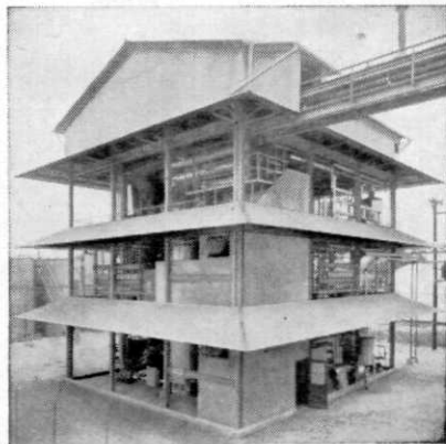
PROCESSING —Allis-Chalmers built solvent extraction plant processes one hundred tons of rice bran per day at oil processing plant in Texas.
