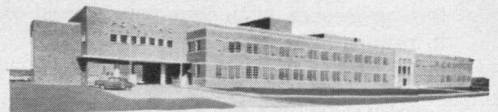
Pontiac's huge new engineering building is the industry's most modern with every conceivable facility for designing better and better Pontiacs.
