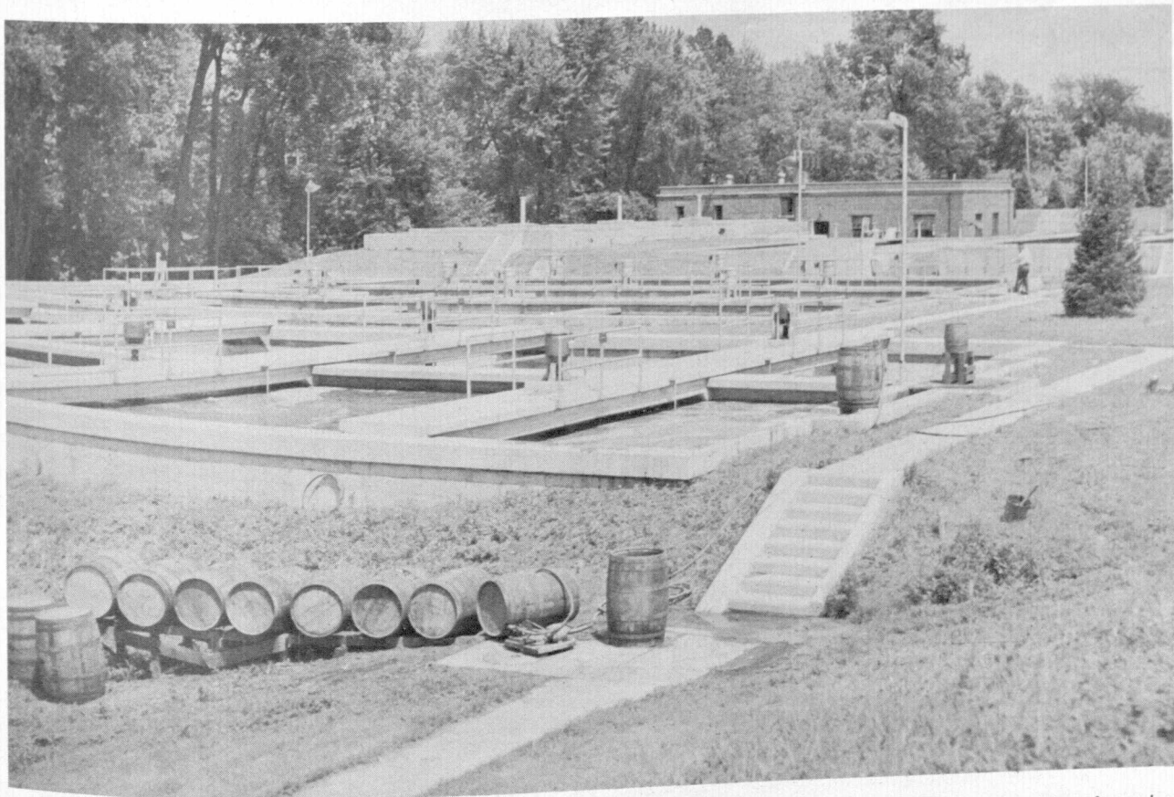
The East Lansing Plant showing the Header Boxes feeding Pickling Liquor to the Aerators.
