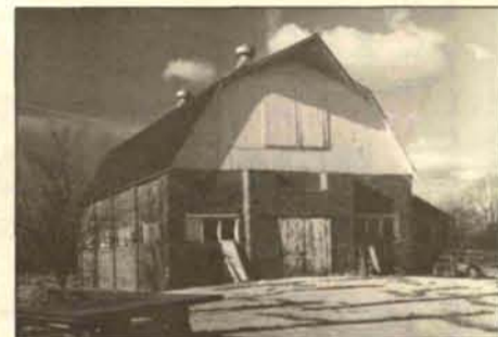
Brick Barn — (southeastern Michigan) Built in 1905-06, the owner of Clippard Brick Works made his barn from the same bricks which paved the streets of Detroit.
