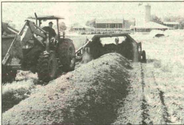
Ionia County Farm Bureau member Ken Gasper demonstrates his push-type compost turner at a field day held on his farm by MSU Extension. Gasper turns his compost piles once a week for six weeks until the process is complete.
