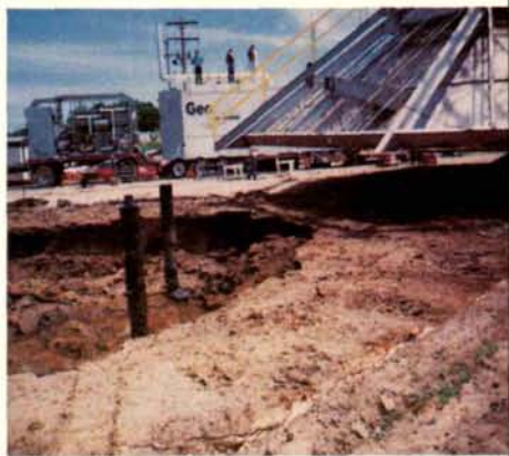
Below, once the melt is completed in an individual cell, the hood is lifted by a crane to the next adjoining cell. The molten soil and the hole left by the melt is backfilled with clean dirt and seeded once the ground has cooled.
