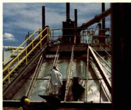
Workers enter the hood to lay down a layer of graphite in a path between four electrodes to start a flow of electricity down into the ground that will melt the contaminated soil. This was the first ever commercial application of "ISV" technology.
