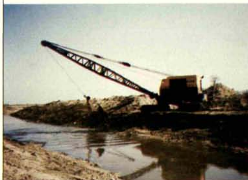
The contractor for the Philp Drain improvement project puts the finishing touches to the drainage bank's contour.
