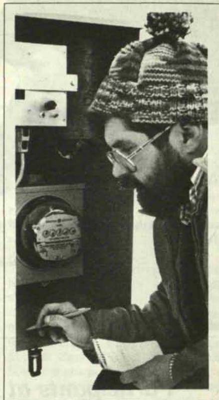
Meters on the Amon farm record wind variables and keep track of kilowatt hours sold the utility company.
