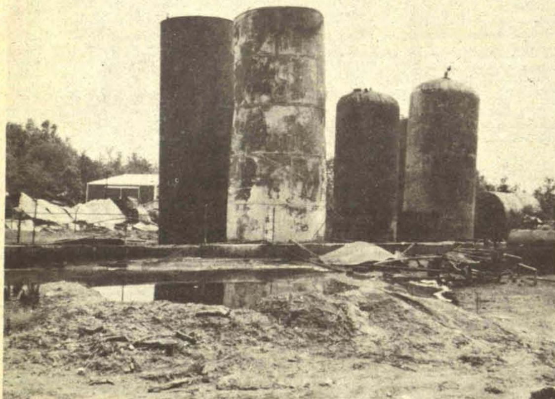
Eight storage tanks, pumping station and 69,000 gallons of fuel were lost in a fire and explosion at Washtenaw Farmers Oil on June 26.
