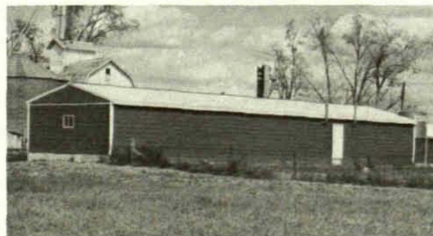
Environmental confinement buildings.
