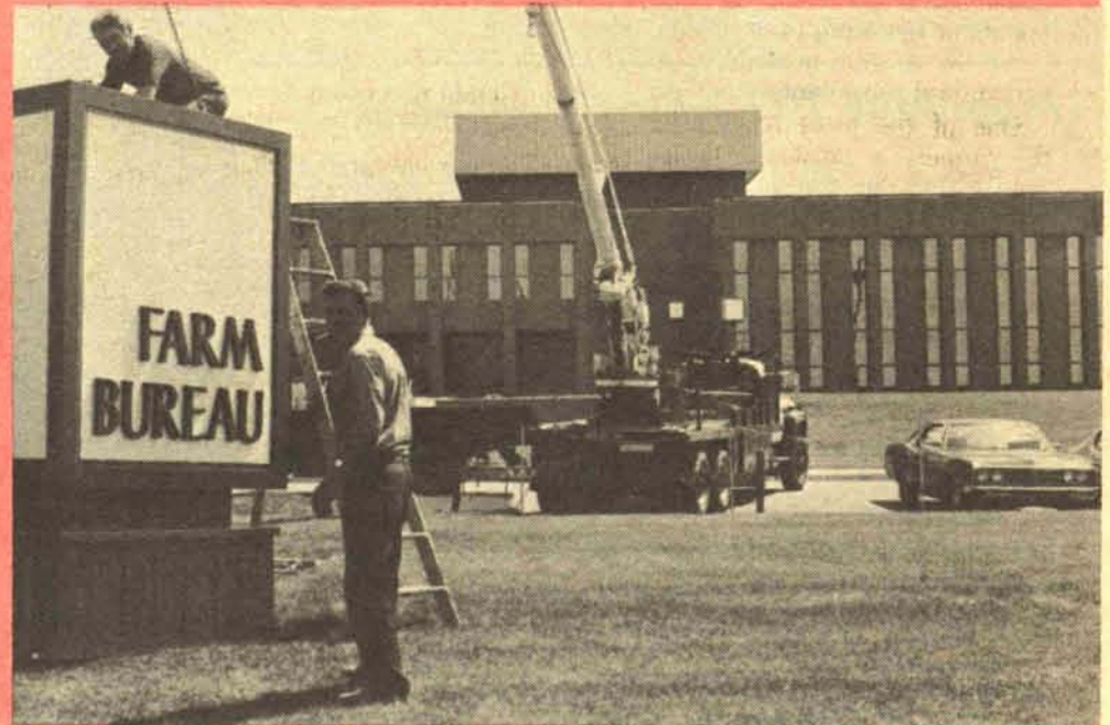
A cubical sign identifying Farm Bureau Center is shown being erected. The design of the frosted lucite, bronze-tone anodized aluminum sign follows the design of the Center and was designed by Norman W. Goodling, MFB.
