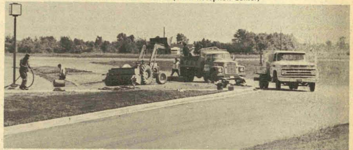
The Laying Down of the Sod
