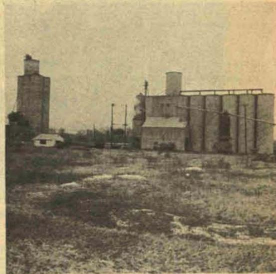
STORAGE COMPLEX — east of Charlotte, holds grain and beans for the Eaton Co-op. Steam pours from the 1,000 bushel per-hour grain dryer. A cluster of "unit-poured" concrete silos for bean storage is part of the complex.
