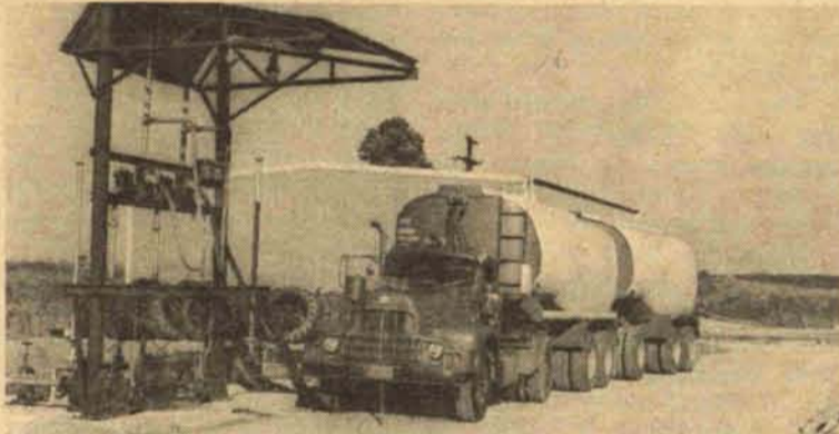
75,000 GALLON underground storage supplies the new plant and tankwagon.
