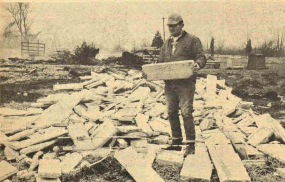
SCRAMBLED SILO — inspected by Tom Adams, Hillsdale. The tornado ripped the roof off their home, disintegrated several farm buildings, scattered 200 bales of hay over the countryside and left this pile of rubble where the silo formerly stood.
