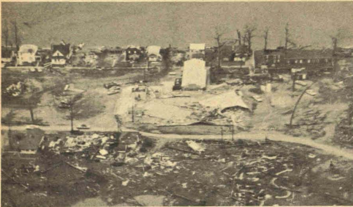
AERIAL PHOTO of the Manitou Beach area in Lenawee County shows a flattened dance pavilion (center, light area). The night before the storm, several hundred teenagers attended a dance there. High as the death toll was (nearly 50 persons in Michigan) — experts agree that many times that number could have been killed.
