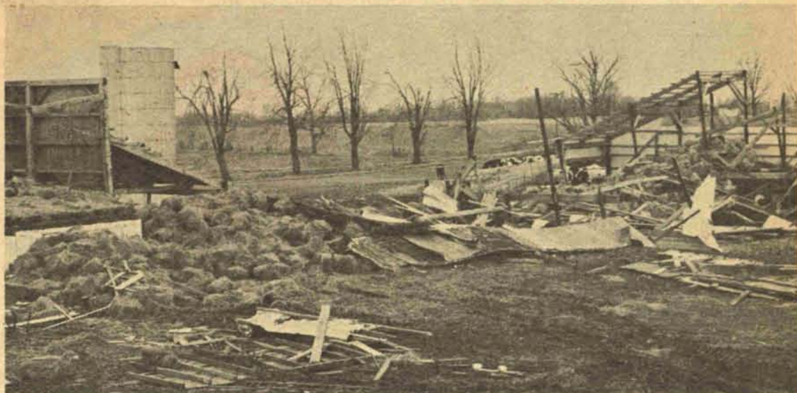
SCATTERED WRECKAGE — a typical sight in parts of Michigan following the Palm Sunday tornadoes. This litter is all that remains of three barns on the Alton Brooks farm in Lenawee County. Although damage was severe, the Brooks considered themselves "lucky." Their home was only slightly damaged, and only one animal was killed.
