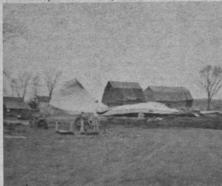
The largest of Anderson's barns, which was about 150 x 40 feet, was knocked off its foundation and completely caved-in by the violent wind.
