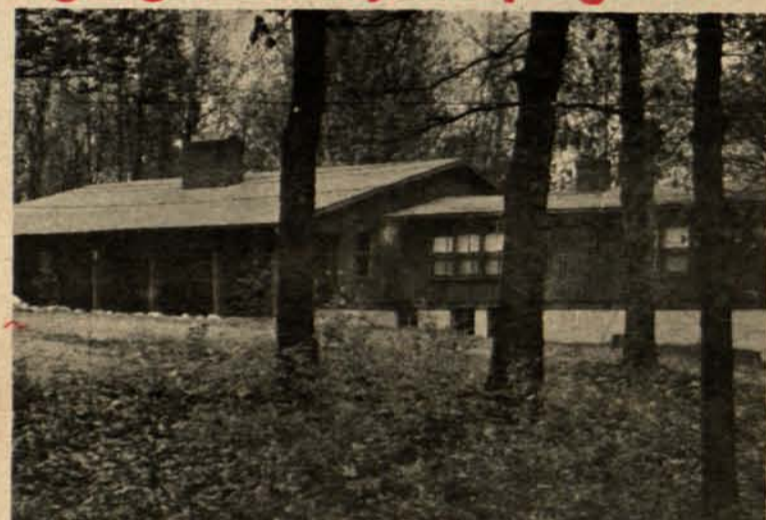
HOLIDAY CAMP for Farm Bureau Women will be held at the Wesley Woods Methodist Camp on Clear Lake near Battle Creek. Shown is the main lodge of the camp site where the two-day event, April 1 and 2, will center around a rural-urban theme.
