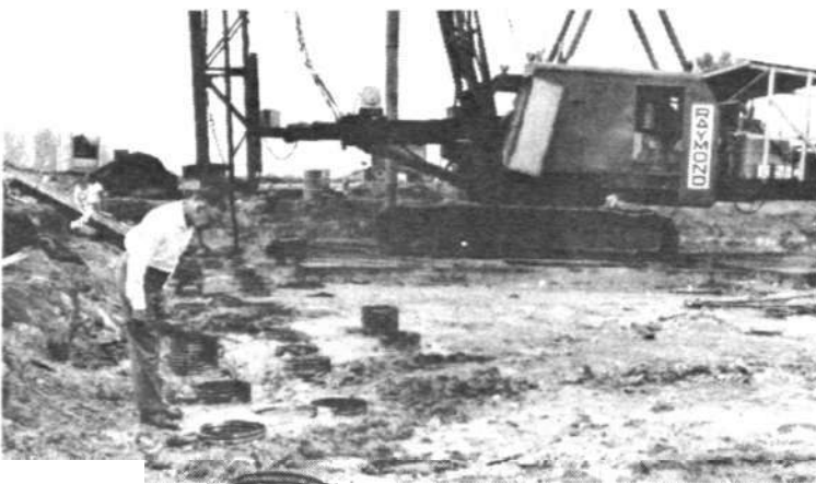
F.B. SERVICES BOARD MEMBER, Max Hood, examines one of the several hundred pilings that will give a firm base to the new grain-terminal near Saginaw. Driven more than 70 feet until "refusal" the hollow pilings are filled with concrete. Work is moving smoothly on the vast project which includes a new feed mill.
