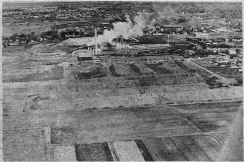
TO KEEP THE MOUNTAINS OF BEETS COOL, the storage piles are "air conditioned"—air ducts are placed laterally at the bottom of each pile and high capacity fans operating during the evening hours circulate cool night air through the beets.
