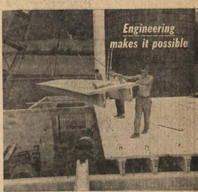
Prestressed concrete double tee units in this barn span 36 ft. The tees are set in place directly from the delivery truck.
