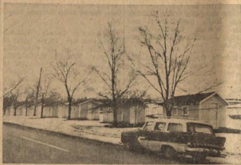
CABINS for migrant workers on the Robert Seeburg farm on the peninsula north of Traverse City.
