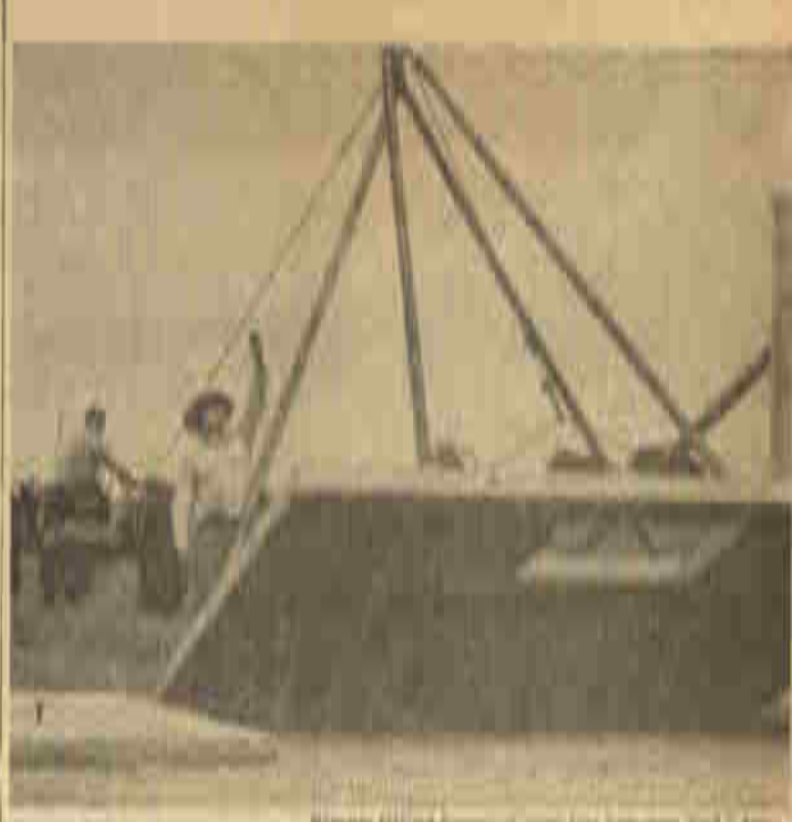
Farmer using "tilt-up" method to set concrete for a structure. The large concrete blocks are set in place.
