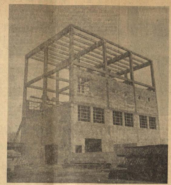
SKELETON-Part of the reinforced concrete framework of the Michigan Farm Bureau seed processing plant remains visible through open areas not enclosed by concrete block walls. Heavy equipment will be suspended from the pre-cast concrete joists, which will support a concrete poured roof. (State Journal, Lansing, photo).
